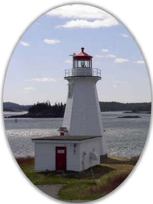
Green's Point Lighthouse
